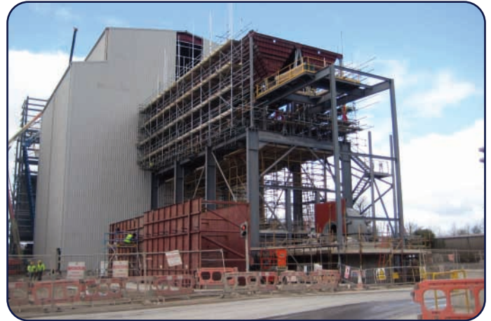
Alongside the cement mill building, the new bag filter housing takes shape. The new bag filter is designed to ensure dust emissions meet stringent EU particulate emission limit values.
