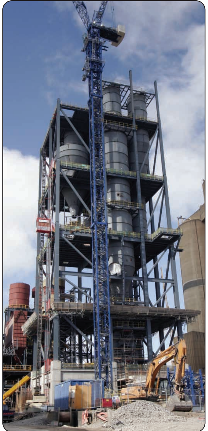
Preheater Tower, now two thirds complete
