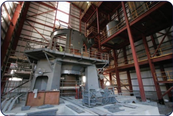
Within the cement mill building, construction of the modern vertical roller mill proceeds. The mill is designed to minimise electricity consumption in the energy intensive milling process, where clinker from the kiln is ground with the addition of gypsum and limestone. The new mill will give Platin the opportunity to maximise the use of limestone, thus producing 'green' cements with a reduced carbon footprint.
