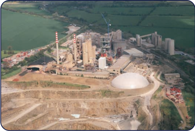
A recent overview of the Platin site. The domed limestone store, which was completed earlier in the year in the foreground is now being commissioned.
