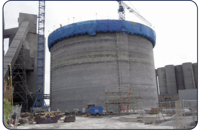
During April, the new concrete clinker silo was constructed by the continuous slip form method of construction. This photo shows the 'slide' nearing completion. Superb finishes on the concrete were achieved by attention to detail in mix design, placing and compaction as the walls were cast.
