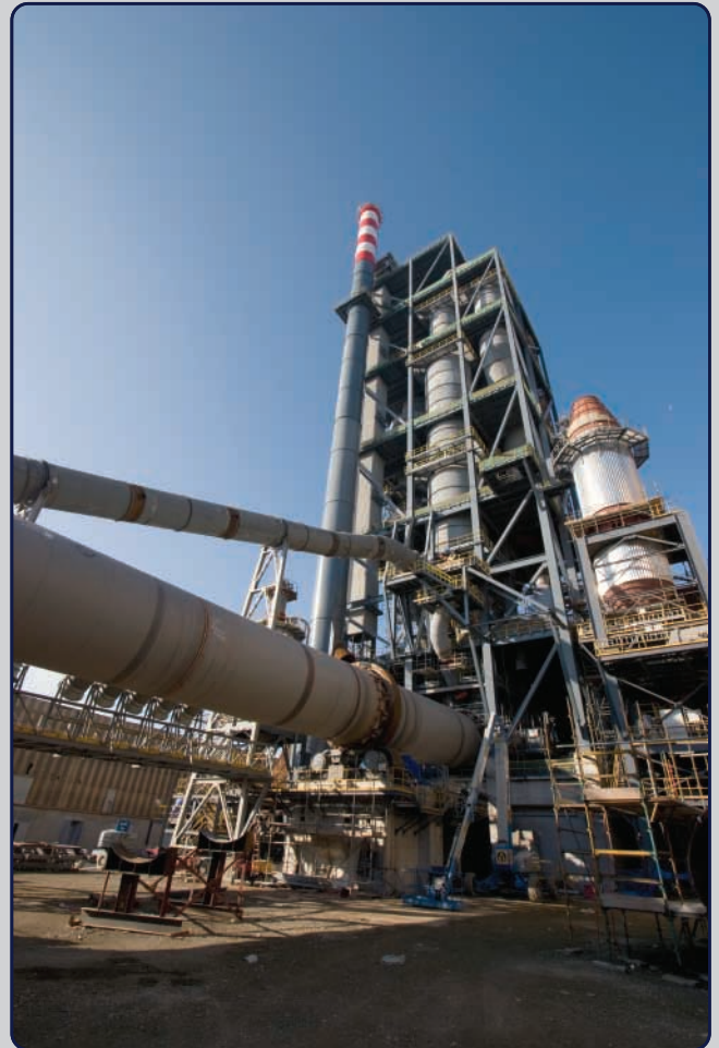
The kiln is now in place and connected to the base of the preheater tower. The technology on-site makes Platin one of the most energy efficient cement plants in Europe with the lowest carbon emissions.
