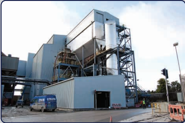
Kiln 3 in Platin will operate to world-class emission standards because of the installation of state-of-the-art bag filters. The bag filter seen here is part of our new energy efficient cement mill 4.
