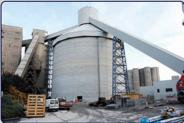
The new clinker silo designed to store 80,000 tonnes of clinker is currently being commissioned. The cooled clinker coming from the kiln is stored here before being transferred to the mills for the final phase of cement production.
