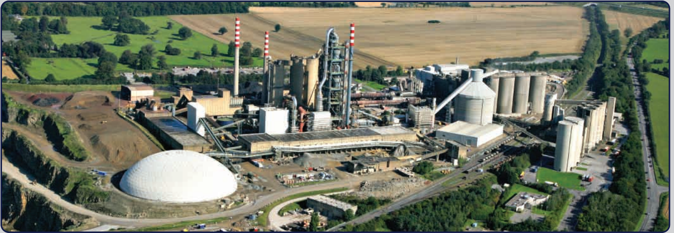
A recent aerial photograph of Platin as the Kiln 3 project nears completion.
