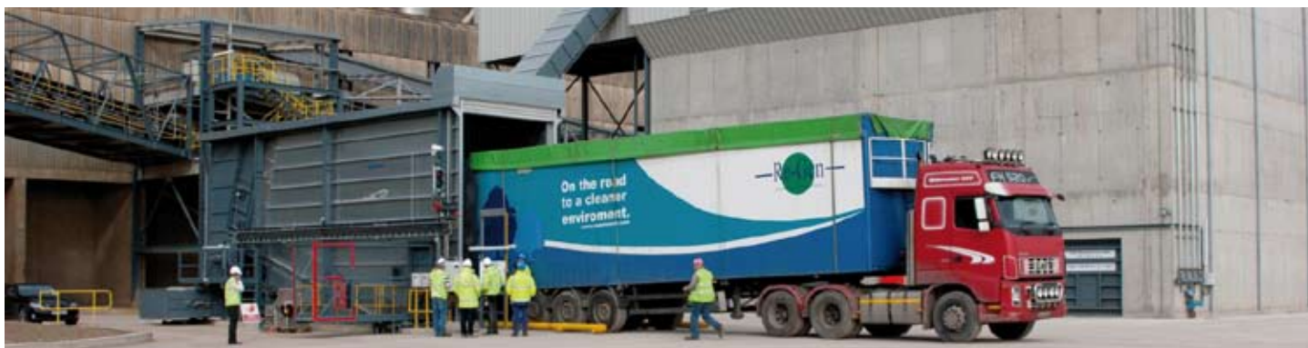
The new truck unloading dock for the alternative fuel store at Platin, receiving its first load of SRF.
